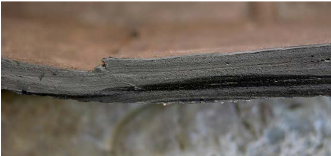
Figure 4: Cross-section of a joint of the membrane
